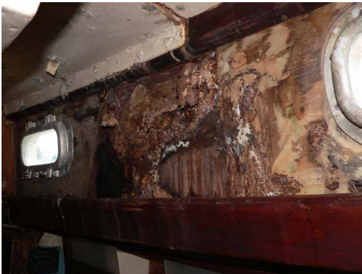
Rotten wood on the coachroof side of salon
